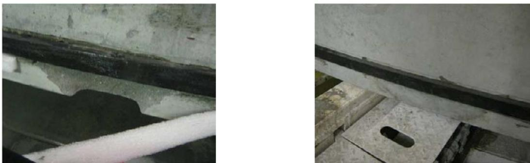
**Figure 6. a) Concrete cover damage detected before installation b) Segment after repair**
